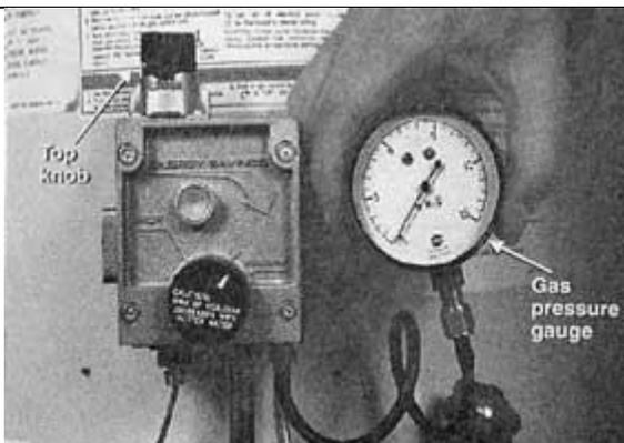
Test gas pressure, bleed air out of gas line
