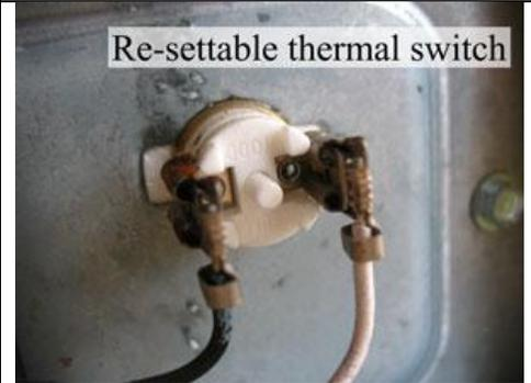
If ECO thermal switch is tripped, burner will not operate
